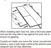
13 Helpful Hint / Consejo clave When installing each new row, take a full loose plank and use the long side to tap against the prior row to ensure no gapping.
